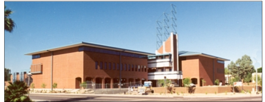
One month before occupancy. The parking lot is fenced for paving and the signage proclaiming the facility as the BLM National Training Center has yet to be added to the face of the 2nd floor elevator walkway. July, 1994.
