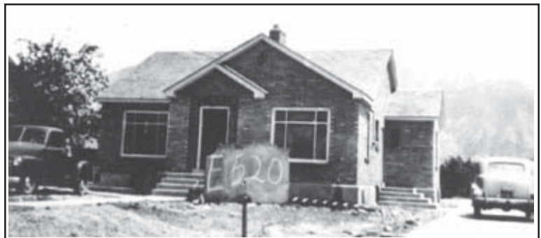
We lived in the basement until the upstairs was completed.
